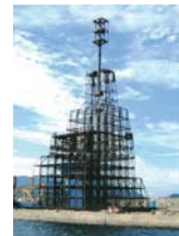
Design and construction methods of high-rise artificial fish reef
